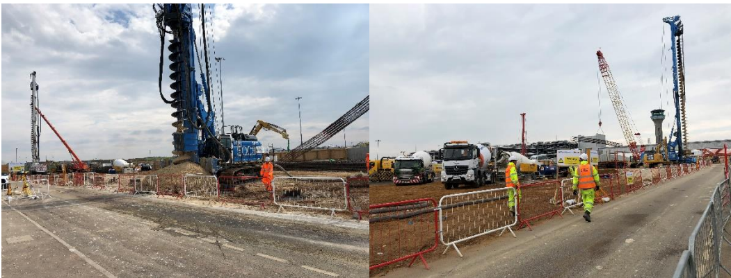
Inset 5.8: Typical CFA piling operations
